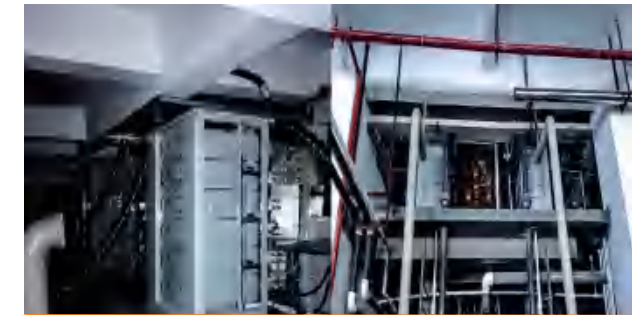
New energy-lithium copper foil Synchronous rectifier-60KA
