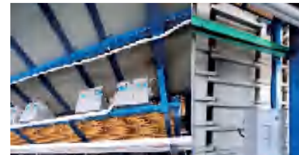
Hydrogen production field Synchronous Rectifier -3000A/12V
